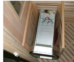
connect the power supply line of stove
